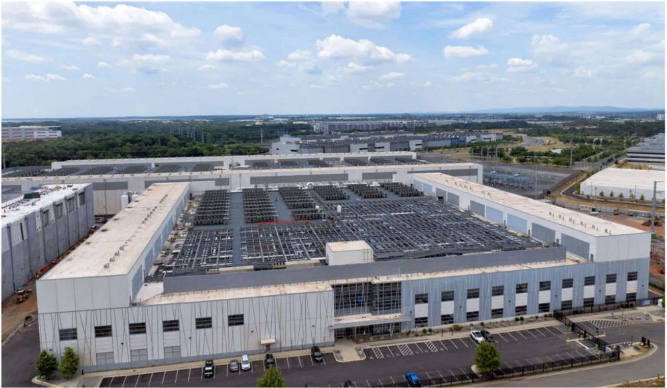
Figure 4 — One of Meta’s three sprawling AI-optimized data centre campuses in Virginia (foreground and background). It currently operates twenty such centres across five countries, with plans for many more. Credit: Meta.
